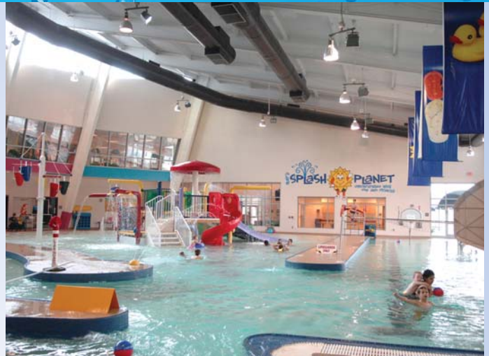
Aquatic centers face differing evaporation levels depending on the occupancy.
